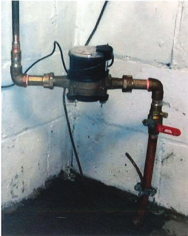
EXAMPLE OF METER SERVICE LINE (SEND IN WITH CHANGE OF OWNER/FINAL READING REQUEST)
